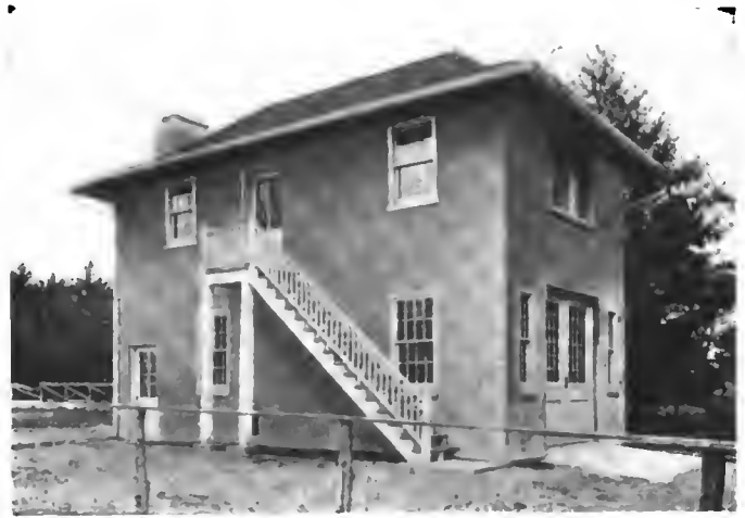
Two-Story Garage of Terra Cotta Hollow Tile Construction
